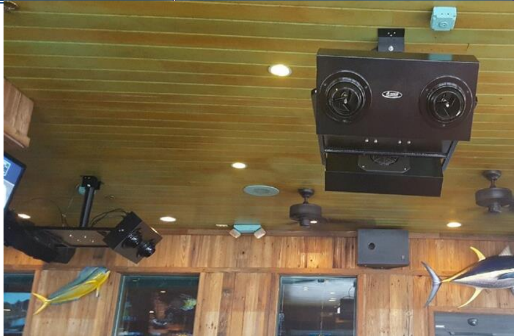
Leah Mounting, Via 2" by 3" Angle, With hole in center of 2 7/8" Diameter pipe to run all power cords, low voltage and misting tubing thru.
